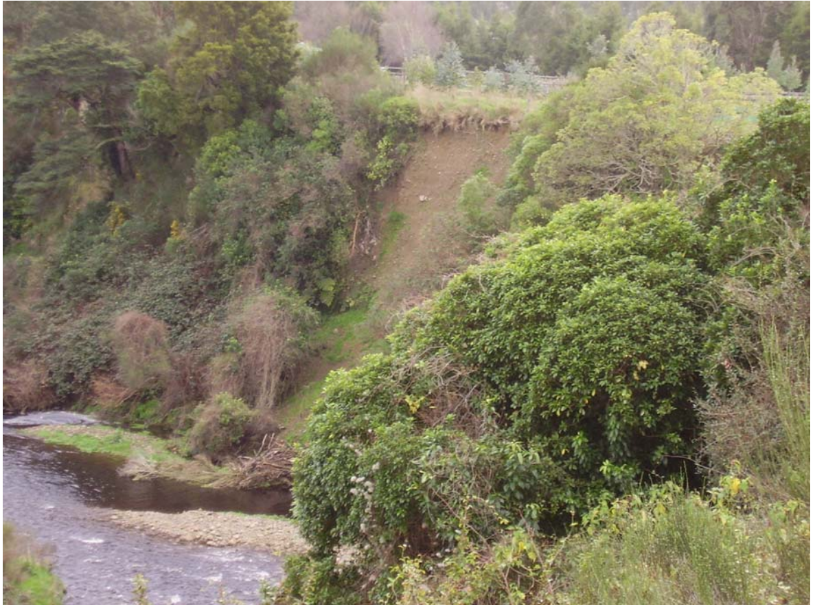
■ Figure 4 River Banks adjacent the Parkes Road.
