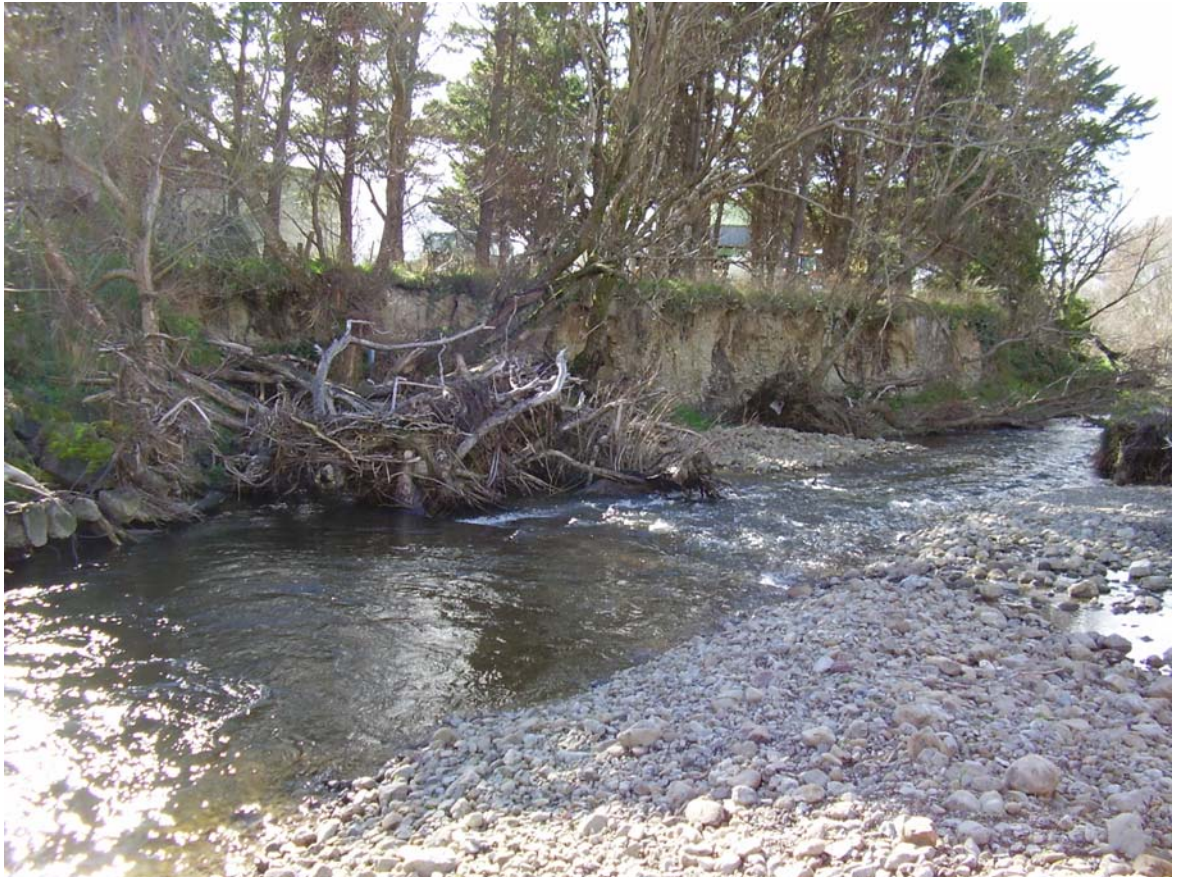
■ Figure 6 Erosion of the Banks Near Mangaroa Valley Road.
