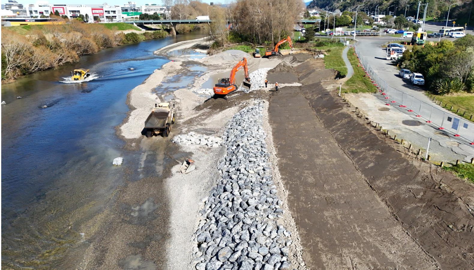
Rockline construction to protect vulnerable river edges and maintain channel performance.
